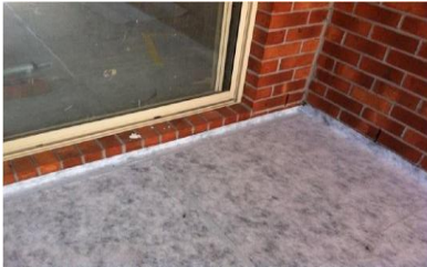
Application of Inoplast PL
